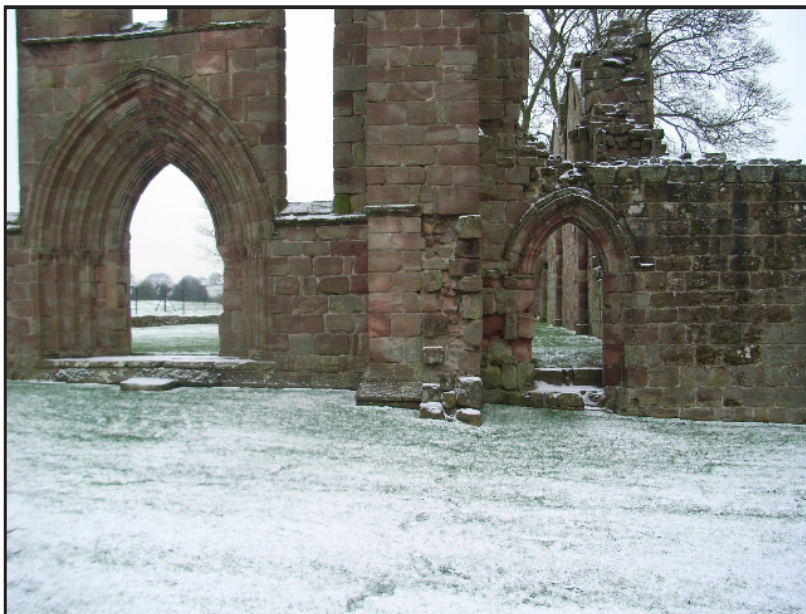
Figure 29. West front of the church showing the position of the wall cut into the south buttress.
