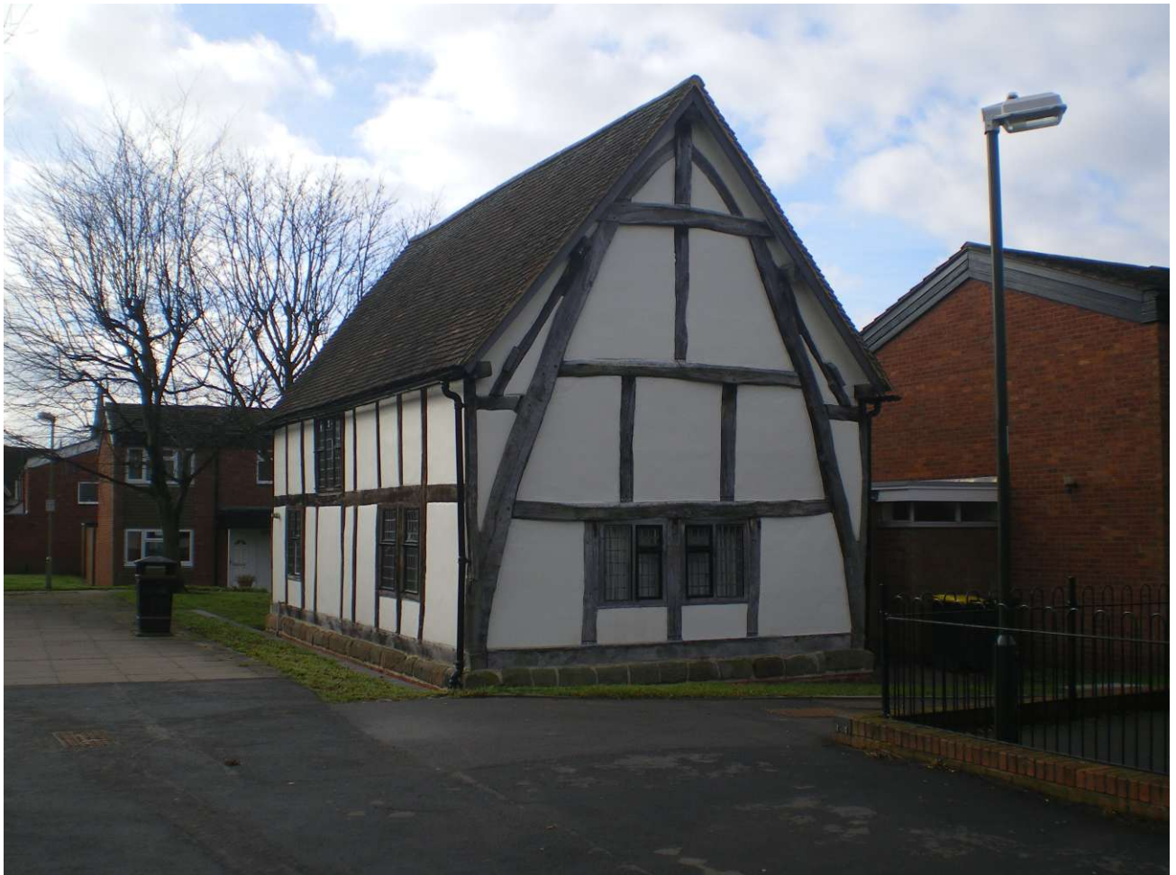
Plate 30: Cruck House, Stowe Street
