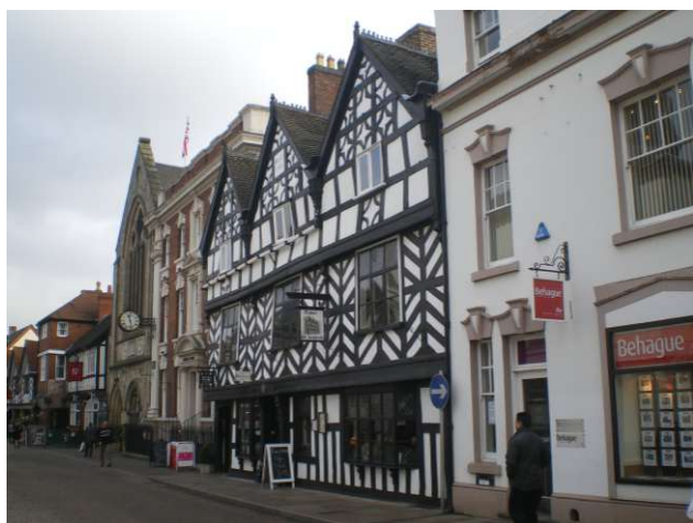
Plate 13: 32 Bore Street – dated to 1510, but probably of late 16th century date
