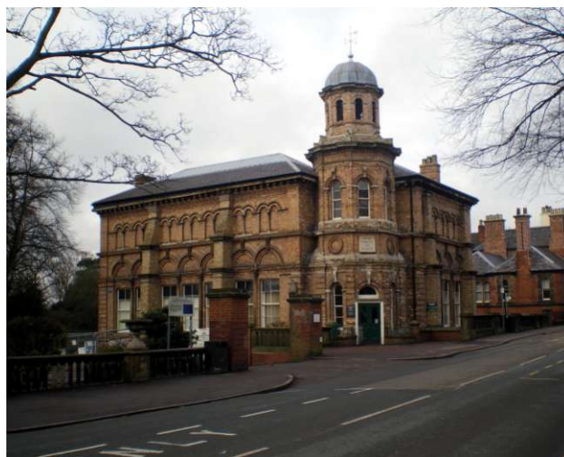
Plate 18: Former public library and art gallery, Bird Street
