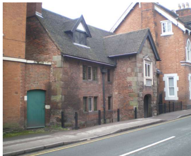
Plate 15: Dr Milley's Hospital, Beacon Street
